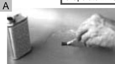
**4** Apply a thin coat of Vyna-Bond adhesive to both surfaces and allow to dry 3 to 10 minutes.
